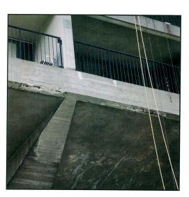
Constructed of cast in-place concrete 30 years ago, this 1200-unit high-rise apartment complex in Fort Lee, New Jersey showed extensive cracking and spalling on the concrete cover of each of its six buildings. Although patch repairs had been carried out periodically, there were continued signs of deterioration.
