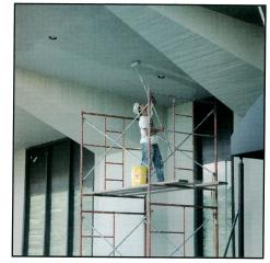
The Sika system specified by Feld, Kaminetzky and Cohen called for the use of SikaTop® repair mortars with Sikagard® Elastocolor, an anti-carbonation, protective coating. With a documented record of long-life protection, this customized combination of Sika products will keep Horizon House healthy for many years to come.
