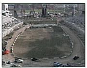
In the midst of renovating the 75-year-old landmark football stadium, it was noticed that the original concrete columns contained no hoop reinforcement. Current code requirements required the use
