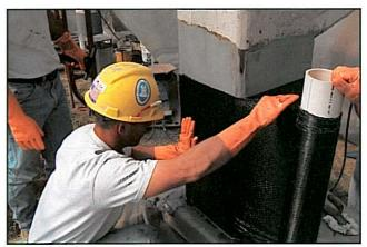
ably light and easy to work with. It is also non-corrosive and requires little to no maintenance once installed. A multiple layer system was installed to meet the structural requirements of the project, yet it remained unobtrusive and was able to be installed even in areas where two columns were only inches apart.
