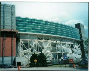
Sandstone was applied to 3 towers of the stadium to provide an aesthetic look. Hundreds of sandstone blocks were applied to the facie of the towers, which also meant that there were thousands of linear feet of joints that needed sealing to prevent water intrusion to the core of the structure. It was very important to the University of Utah to maintain the sandstone color throughout the entire surface and not have any staining take place that would degrade the appearance.
