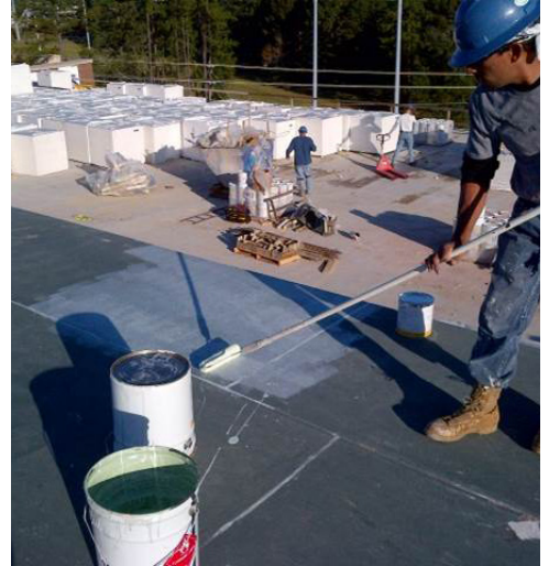
Step 6 - Surfacing/Overburden**
