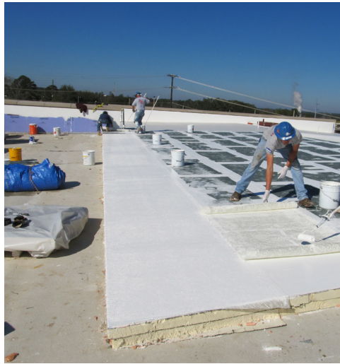
Step 4 - Membrane Application
