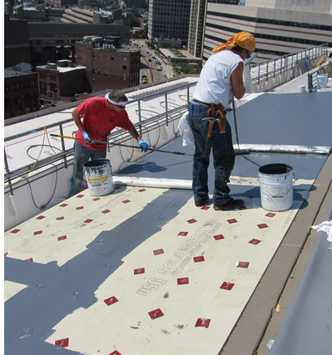
Step 4 - Membrane Application
