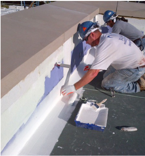
Step 4 - Detailing/Flashing
