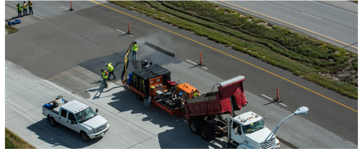
High Friction Surface Treatment (HFST) is a single layer epoxy application with high friction aggregate that significantly and immediately increases roadway friction to reduce auto crashes, injuries and fatalities on problem road surfaces.
