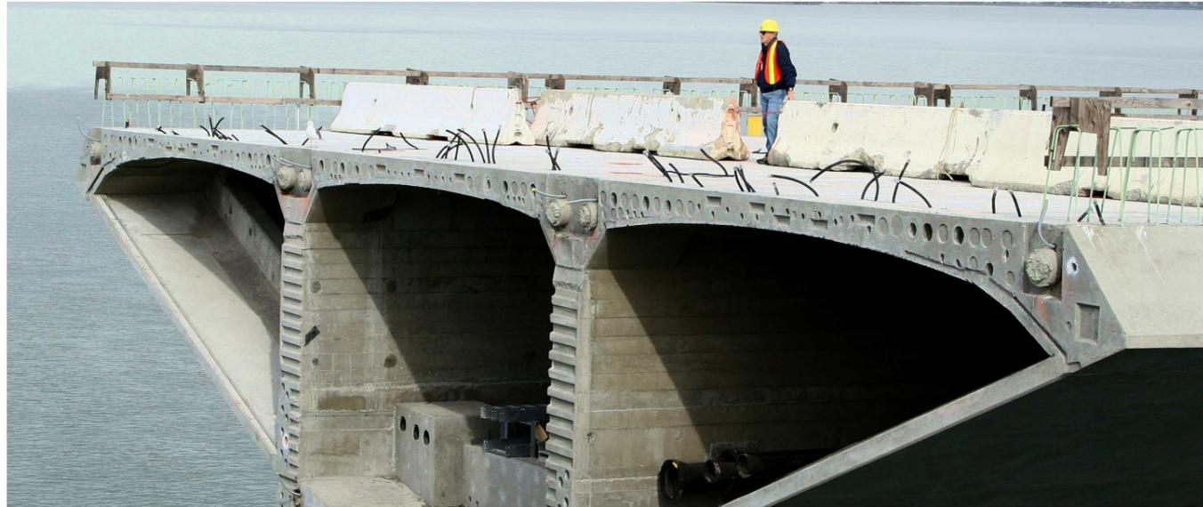
Sika's high-performance epoxy Segmental Bridge Adhesives (SBA) are high modulus, high strength and moisture tolerant allowing for the bonding of bridge segments in specific temperature ranges, from 20°F - 115°F.
