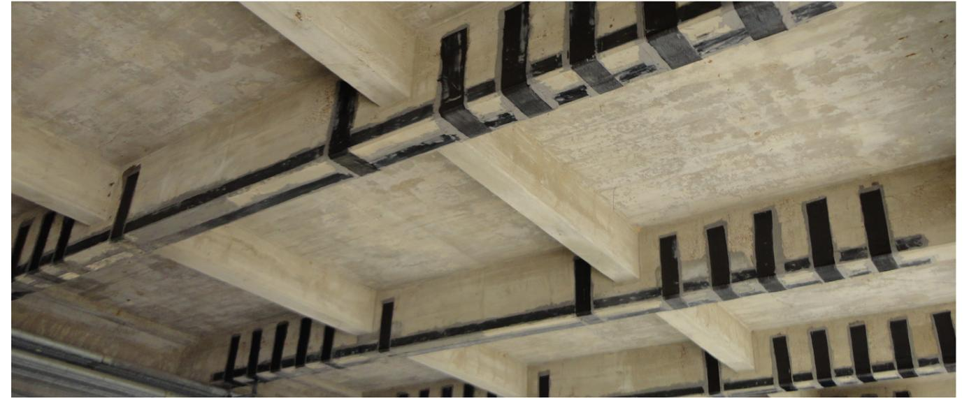
SikaWrap and CarboDur composite materials are constantly used in critical applications to solve challenging structural problems, including but not limited to confinement and shear strengthening, seismic upgrades, impact and blast resistance, and design or construction defects.
