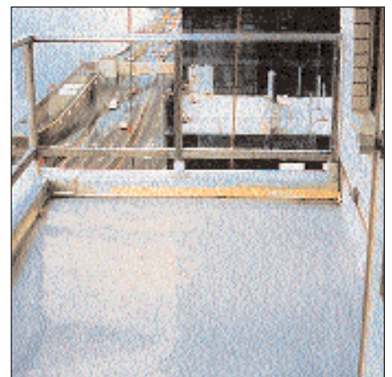
Sikafloor Traffic System on a Private Balcony
