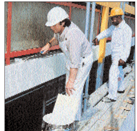
Roller Application of Sikagard Elastocolor
