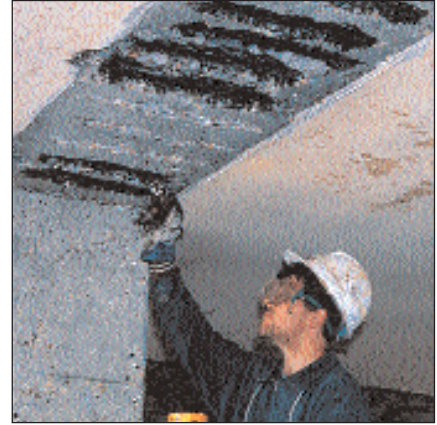
Brush Application of Sika Armatec 110 EpoCem on a Soffit
