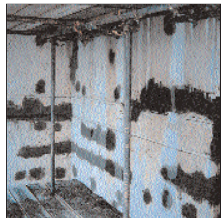
Spalls filled with Sika MonoTop Ready for Leveling and Protection
