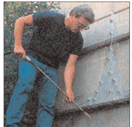
Sikadur Injection System on a Building Facade
