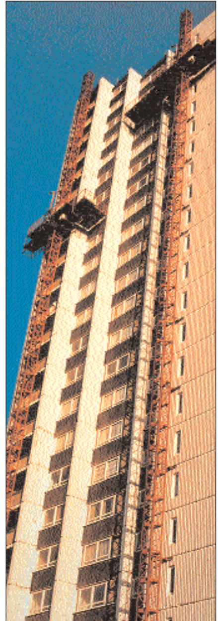
Concrete Repair and Protection Project in Progress
