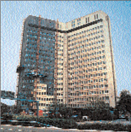
Repair Project in Initial Surface Cleaning Phase
