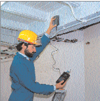
Covermeter Survey to Determine Depth of Steel Reinforcement
