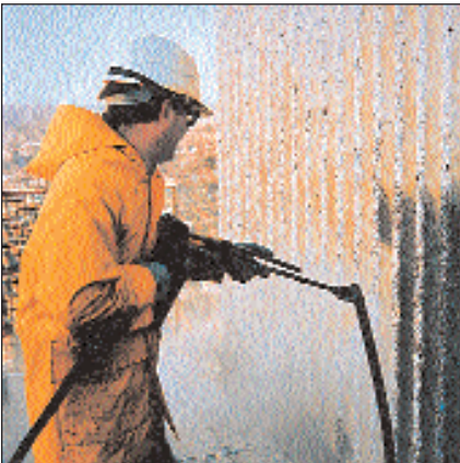
High Pressure Water Cleaning Before Marking out for Repairs
