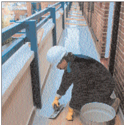
Trowel Application of Sikafloor Traffic System on a Public Balcony
