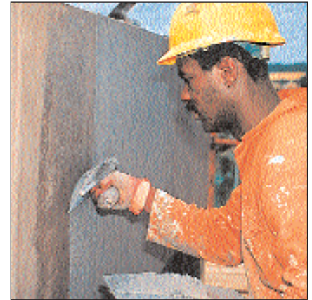
Trowel Application of Sika Leveling Mortar on a Parapet
