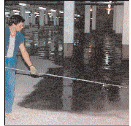
Spray Application of Sika FerroGard 903 on a Parking Deck
