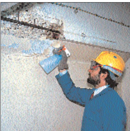
Carbonation Depth Testing with Phenolphthalein
