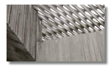
gate sources, admixtures and physical properties of concrete. The trial mixtures and samples evolved into larger mock up samples that were evaluated by the entire construction team for consistency and reproducibility over time on the project. To ensure that the desired consistency and surface finish
