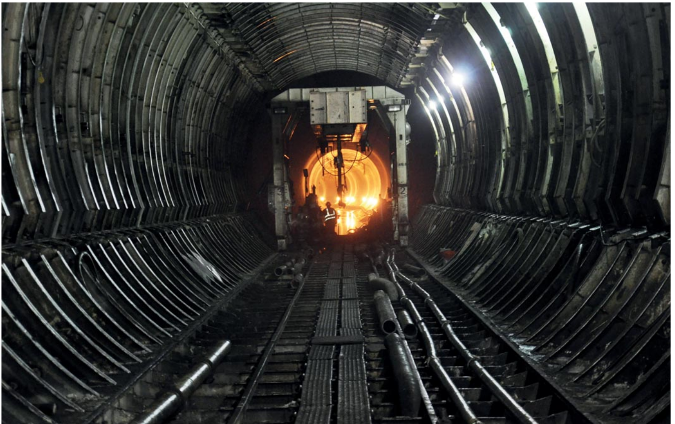
A collapsable forming system coupled with SCC increased speed of construction
