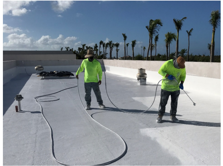
Spray-applying the Sikalastic RoofPro liquid-applied membrane at Four Seasons.
