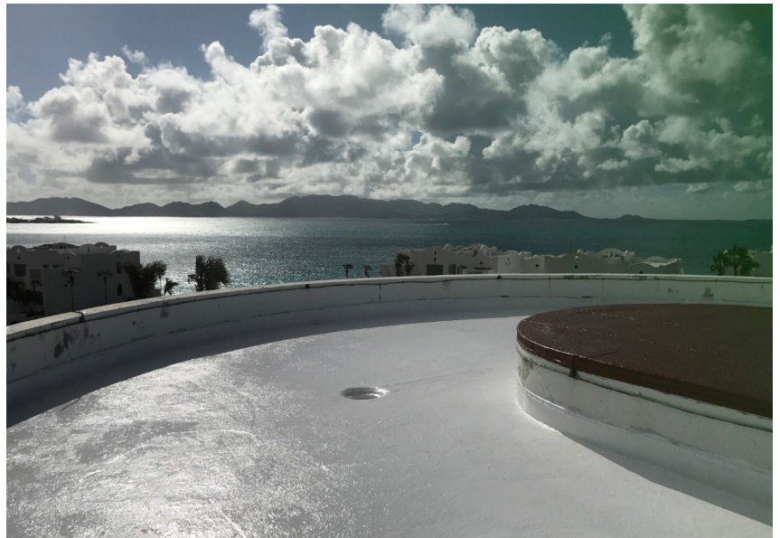
Sikalastic RoofPro membrane at Anguilla's Cuisinart Resort with the mountains of Saint Martin in the background.
