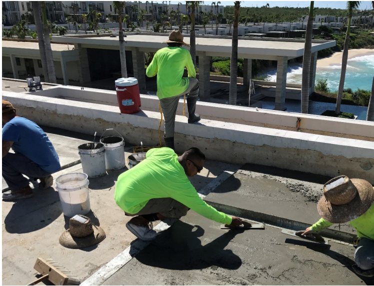
SikaQuick 1000 trowel-applied from 6" to 1/4" in depth was used to slope the concrete roof decks so that rainwater would drain from the flat roofs.
