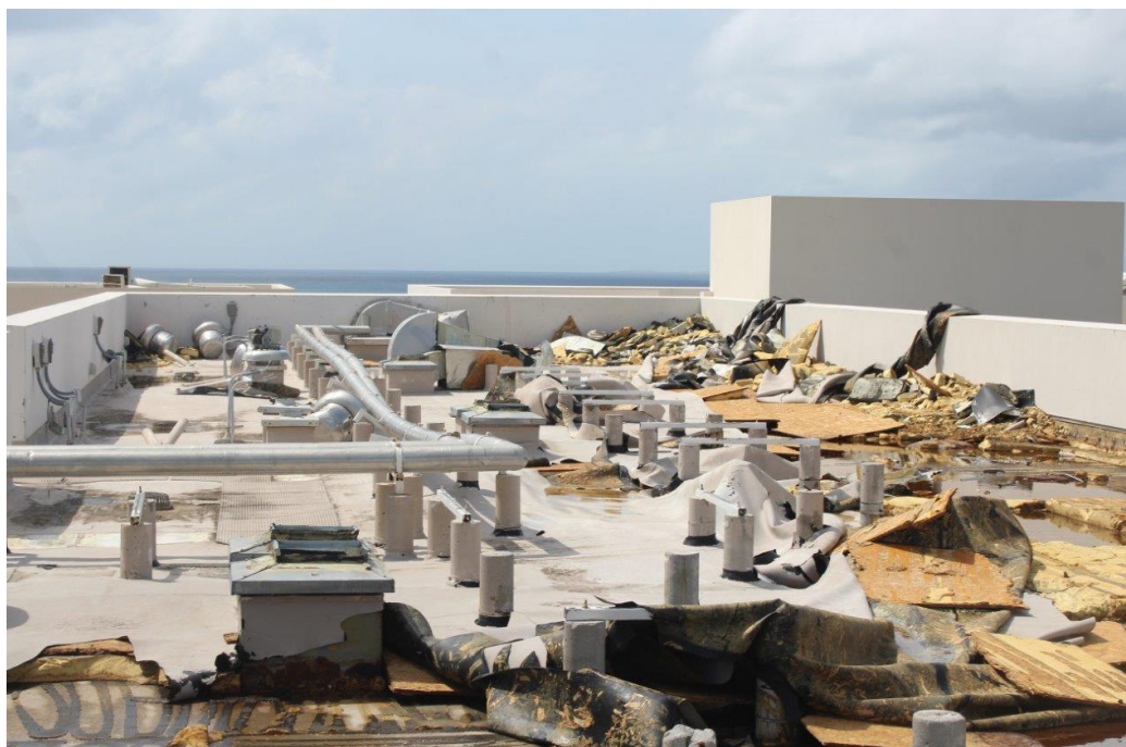
Hurricane damage to EPDM and tapered insulation assembly on roof.
