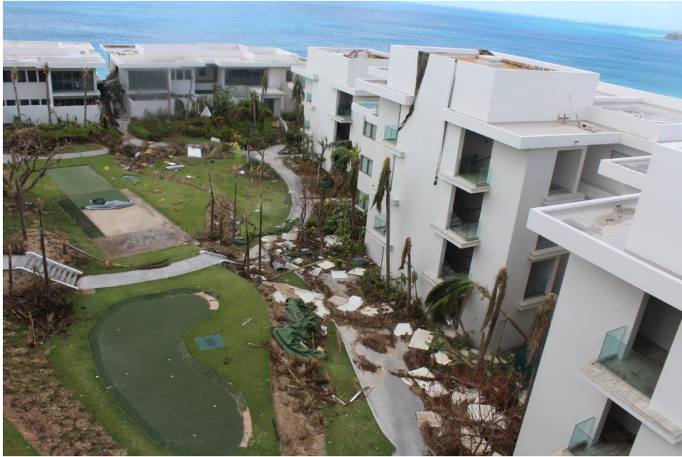
Damage to the buildings at the Four Seasons Resort in Anguilla caused by Hurricane Irma.
