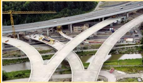
Sika® Dilatec® allows elastic bridging and sealing of construction and movement joints to protect the bridge construction (reinforcement and others).
