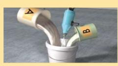
2. Mix Sikadur®-Combiflex® CF adhesive or Sikadur®-31 CF for a minimum of 3 minutes until the mix is homogeneous.
