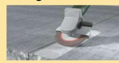
1. Substrate preparation by means of sand blasting, grinding etc., followed by vacuuming.
