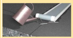
2. Unroll the Sika® Dilatec® strip with the wide fabric B-edge facing up and fix the edges by soaking them with liquid hot bitumen; make sure that the narrow fabric strip is completely saturated.
