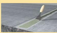
3. In the location of the fabric strips, apply Sikadur®-Combiflex® CF adhesive or Sikadur®-31 CF without gaps (layer thickness 1-2 mm and overlap of 10 mm). For a cleaner edge, an adhesive masking tape can be used and then removed after application (before curing)
