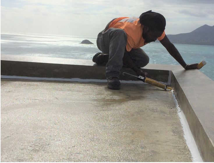
Sikaflex 11 FC sealant at deck to wall joint
