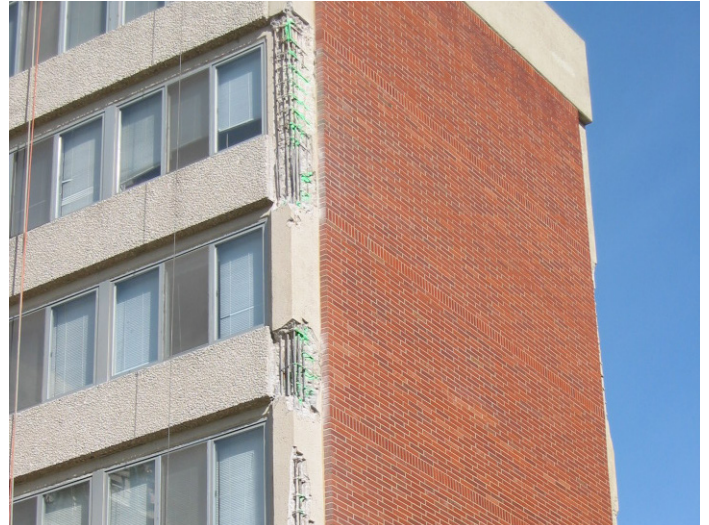
Spalled concrete at columns accelerated by lack of adequate cover
