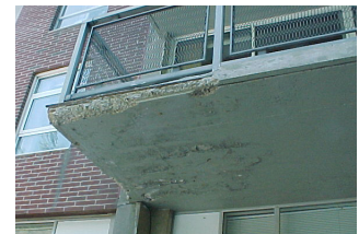
UNDERSIDE & BALCONY EDGE SPALLS
