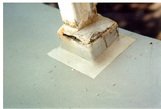
RAIL POST DEGRADATION
