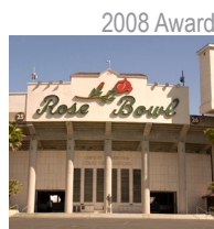
Repaired in 1998 Rose Bowl Stadium Restoration
