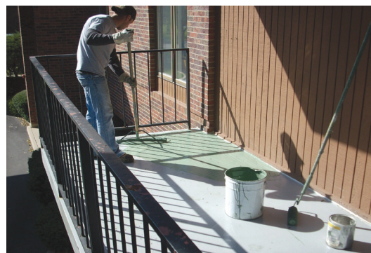
Application of Sikalastic® Seafoam top coat.
