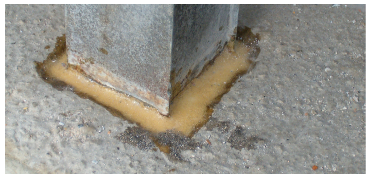
Sikadur ® 21 Lo-Mod with oven dried aggregate for rail post grout.
