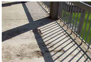
BALCONY SURFACE EROSION
