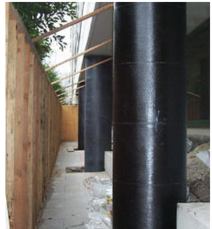
Seismic strengthening of columns with carbon fiber fabrics.
