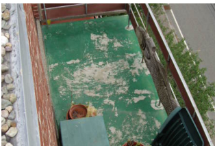
FAILED BALCONY COATING
