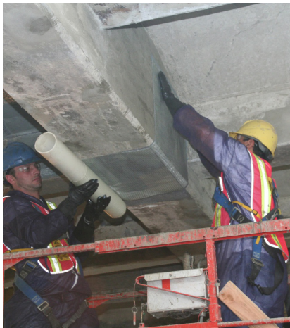
SikaWrap® System used to reinforce a concrete beam.
