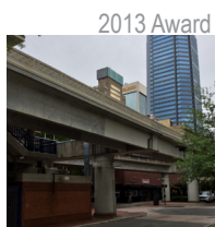
Repaired in 2000 JTA Skyway Restoration
