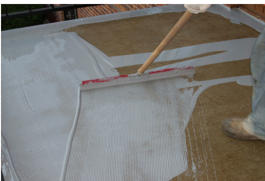
Application of Sikalastic® base coat.
