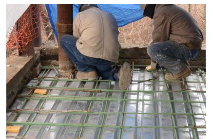
FerroGard® anodes installed where an existing slab and a new, full-depth slab meet
