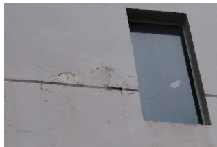
FAILED FACADE COATING
