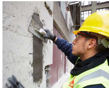
SikaTop ® 123 Plus used for vertical repairs.
