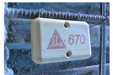
FerroGard® Anodes used to prevent corrosion of rebar near the balcony edge
