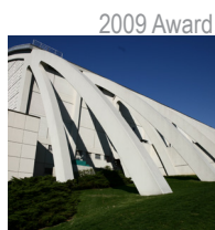
Repaired in 1997 Cassell Coliseum at VA Tech Univ.
