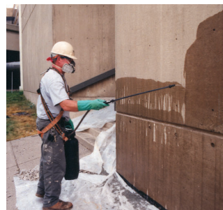
Application of Sika® FerroGard® 903 to a building (l) and a balcony (r)
