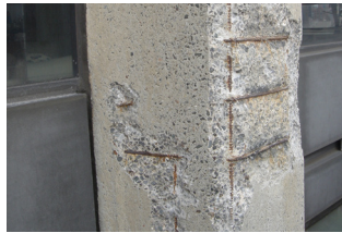
POOR CONCRETE COVER
