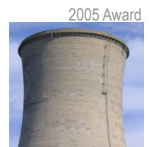
Repaired in 1988-1990 Rehabilitation of Two Hyperbolic Cooling Towers
