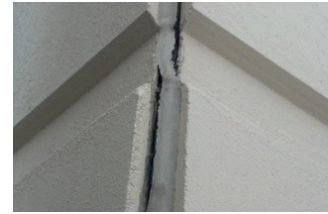
SEALANT ADHESION FAILURE
