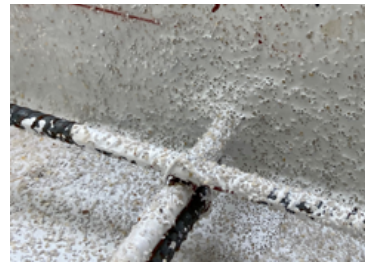
Re-bar Encapsulation
