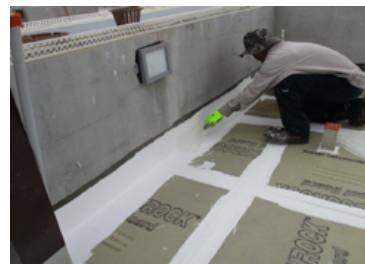
Insulation/Cover Board Installation
