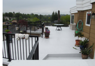
Carports - Roof Decks
