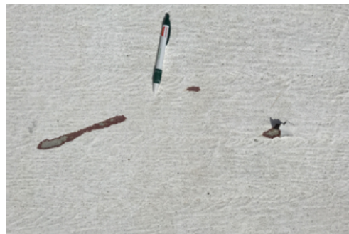
Still bonded after 185 mph winds from Hurricane Irma - only gouges in top of membrane
