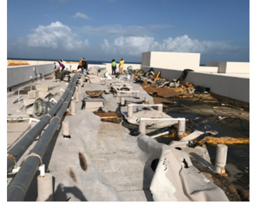
Torn off loose laid membrane system
