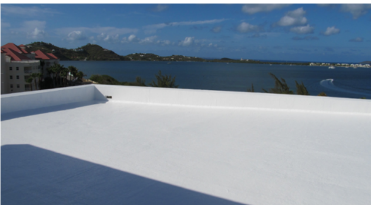
Sikalastic® RoofPro membrane on the medical building roof at the American University of the Caribbean in St. Martin
