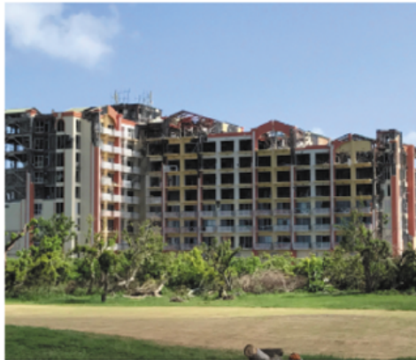
Hurricane damaged building
