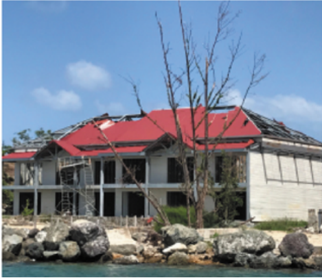
Coastal home with torn off roof
