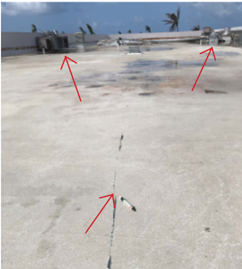
Mechanical equipment that became airborne on the CEP building during the hurricane caused skid marks in the RoofPro membrane
