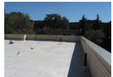
Typical Built Up Finished Roof
