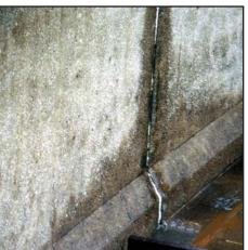
sive water chemistry. Concrete that is exposed to water with a pH of 6 or less, produces new calcium compounds which are very soluble and can easily erode. The presence of low pH water at Andover had weakened, and in many cases dissolved the top 1/4 to 1/2 inch of cement matrix. Ignoring the problem was unacceptable since further erosion of the cement matrix would have necessitated large scale repairs or total replacement within a few years.
