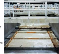
*Sikadur Combiflex* - a unique strip and seal system used to seal problem joints and cracks, even those undergoing extreme movement. Failed joint sealants need not be removed prior to installing Combiflex(a great labor savings.
