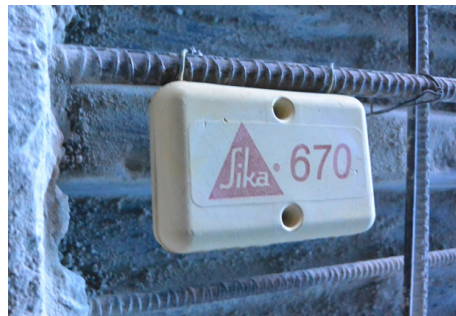
FerroGard anodes installed where an existing slab and a new, full-depth slab meet
