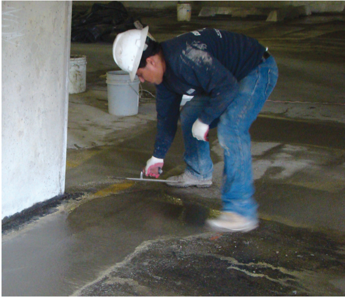
Spall repairs on a slab with SikaTop® 122 Plus
