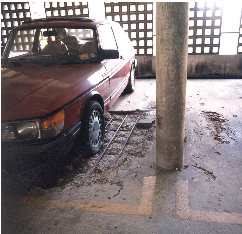
Severe slab degradation
