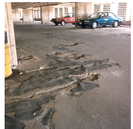
Chloride-induced corrosion causing spalling of the concrete deck
