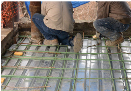
FerroGard Anodes used to prevent corrosion of rebar near the slab edge
