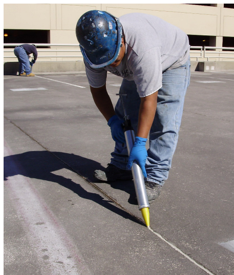
Sikaflex® 2c SL two component, self-leveling sealant applied to joints
