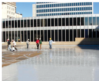
Sikalastic® 710 Base coat application
