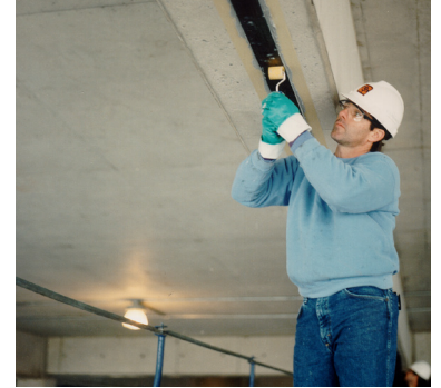
Flexural strengthening of beam with Sika® CarboDur® strips
