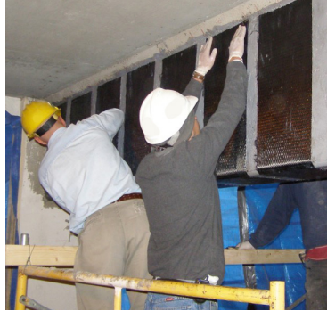
Shear strengthening of beam with SikaWrap® fabrics
