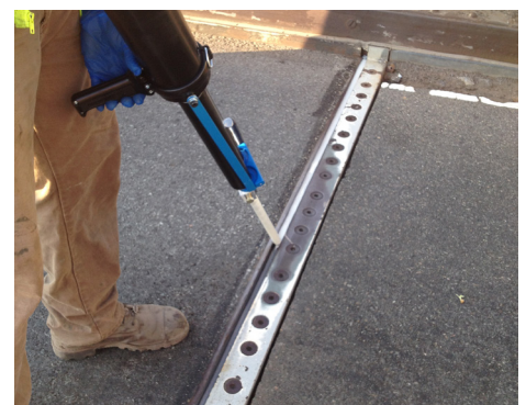
Sikasil®-728 RCS being applied on a bridge deck
