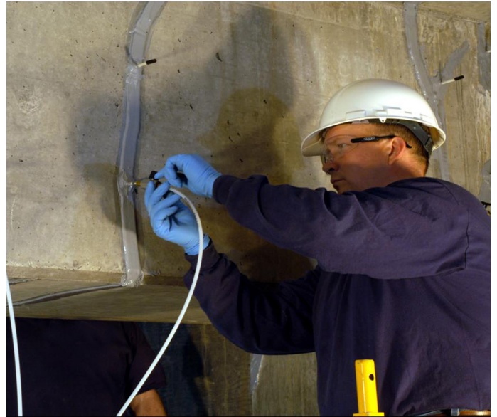
Structural cracks injected with Sikadur® resins
