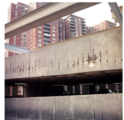
Corrosion accelerated by carbonation and low cover
