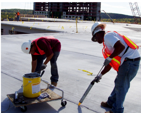
Sikaflex® 2c NS EZ Mix, two component, polyurethane sealant application
