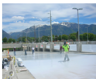
Sikalastic® 715 Top coat application
