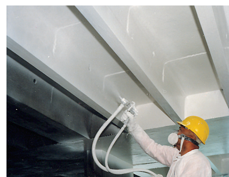
Sikagard® 670W acrylic protective coating spray applied. Excellent option to increase light reflectivity and brightness
