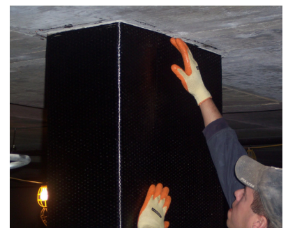
Strengthening concrete column with SikaWrap® fabric
