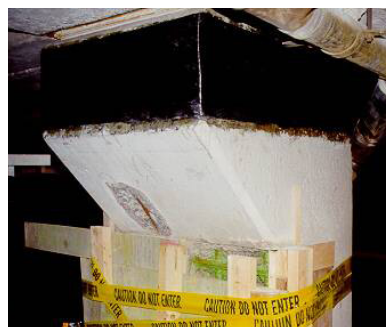
Corbel strengthening with SikaWrap® fabric
