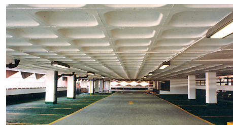
Sikagard® 670W anti-carbonation coating applied to underside of slab/ceiling
