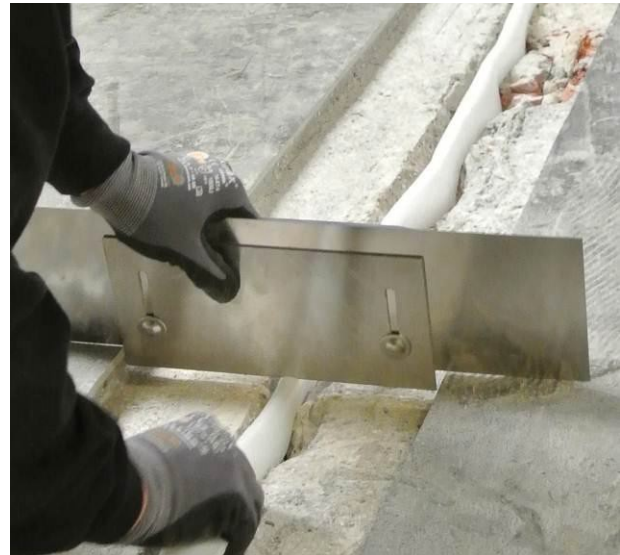
Adjusting the height of the stripping using adjustable trowel
