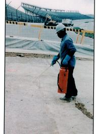
Finally, the surface was leveled with a new concrete overlay. A new waterproofing membrane was applied to the top of the tunnel before the new asphalt racing surface was applied.
