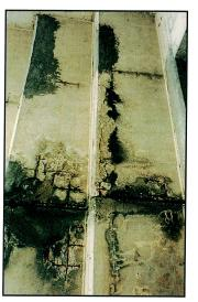
The entire racetrack of this world-famous speedway was being prepared for re-paving. Prior to replacement of the asphalt, six concrete tunnels which served as entry points to the interior of the raceway were inspected and found in need of repair. Corrosion of the reinforcing steel was prevalent, mainly caused by some chlorides and carbonation (pH loss) of the concrete.
