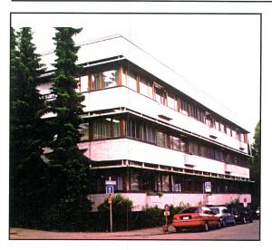
The 3-story office building in downtown Zurich (CH) showed cracks and minor spalls on the concrete elements of the facade. The coating was weathering off and could no longer protect the concrete from deterioration.
