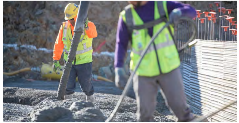
Kiewit Construction placing concrete during the repair process
