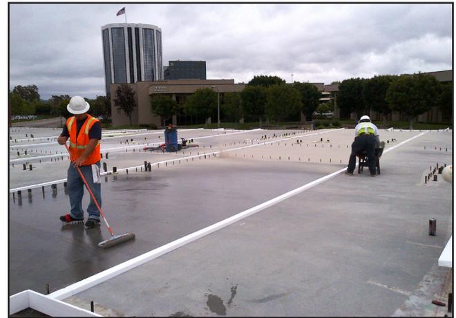
**Sikadur® 32, Hi-mod** – a multi-purpose, 2-component, 100% solids, moisture-tolerant structural epoxy adhesive. It conforms to the current ASTM C-881, Types I, II, and V, Grade-2, Class C and AASHTO M-235 specifications.
