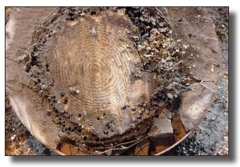
The wood timber piles of the original construction were of green untreated wood which at that time was in vast supply. With the cleanup of the river came the return of the marine life. One such organism were the marine worms that made their home in the piles and also used them as a food supply. They bored holes throughout these piles, detiorating and weakening them. Also noticeable was the fact that the piles were sinking into the mud line on the bottom of the river.
