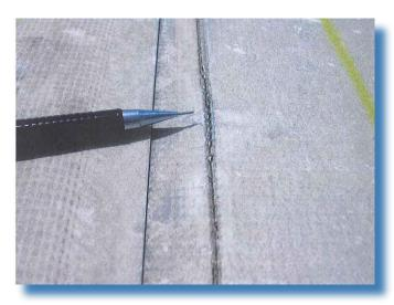
Split of TPO membrane at field seam.
