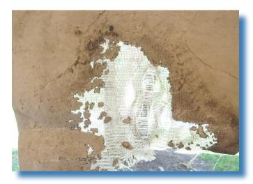
Dramatic loss of TPO polymer, exposing reinforcing scim.
