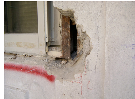
Good example of spalling caused by the window steel flange corrosion.
