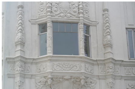
Completed area with intricate detailing and ornamentation. The four vertical elements of the window are made of GFRC.
