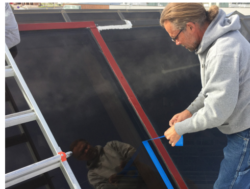
Always pull the tape while the Sikalastic® Clearglaze is wet to leave a clean sharp edge.
