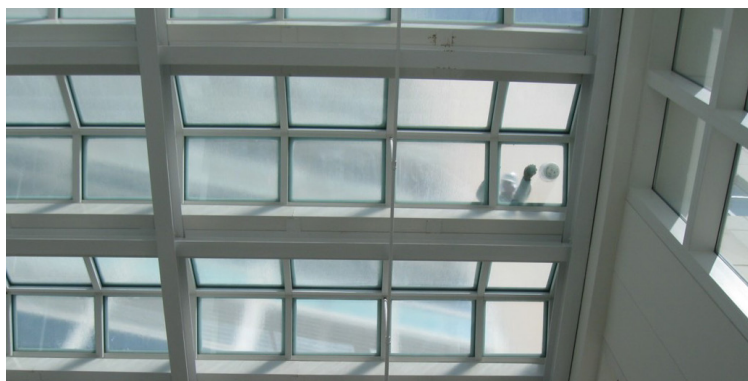
Appearance of Sikalastic® Clearglaze applied to existing skylights
