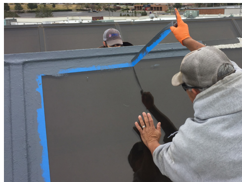
While the Sikalastic® RoofPro resin is wet lay in precut lengths of Sika reinforcing scrim and embed with a wet roller or brush to ensure full saturation and conformation to the substrate.
