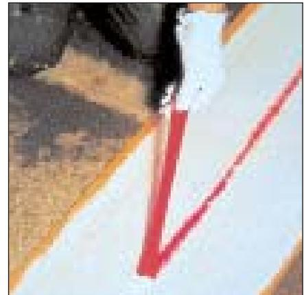
**6** Remove red center strip before *Sikadur 31* fully hardens. **Note: This is best done within one hour at 73°F (22°C). Overlapping sections or details are permanently bonded on or off site using hot weld guns.**
