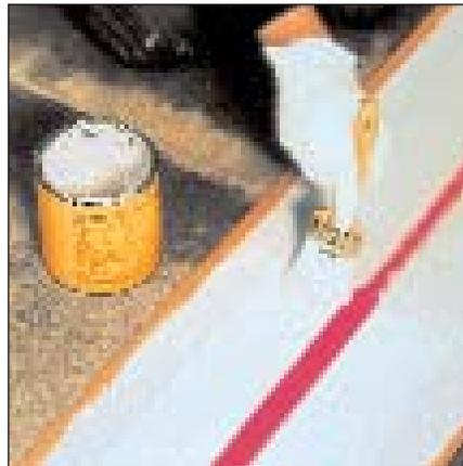
**5** With brush or trowel, apply a top layer of *Sikadur 31* over entire width of sheeting. **Note: Do not deliberately waste adhesive over red center strip.**
