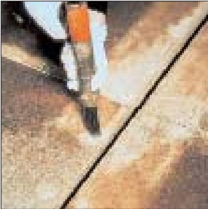
**1** Thoroughly clean the bond surface mechanically. **Note: No need to remove existing failed joint sealant.**
