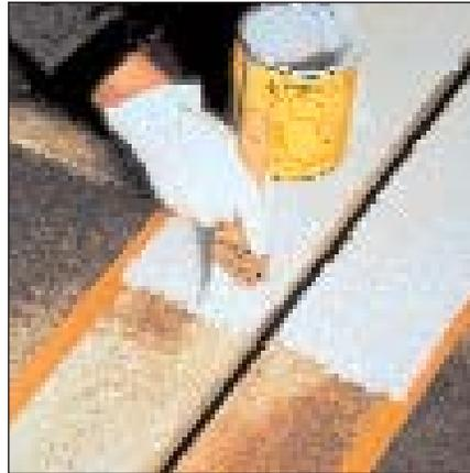
**2** Apply *Sikadur 31* epoxy adhesive by brush or trowel on each side of the joint or crack. **Note: No need to repair all joint nosings.**
