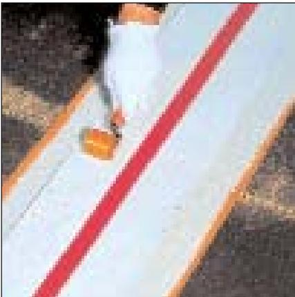
**4** Roll *Sikadur Combiflex* strip to exclude air through the special perforations until adhesive comes through. **Note: Allow sheeting to drape in slot for high movement joints.**
