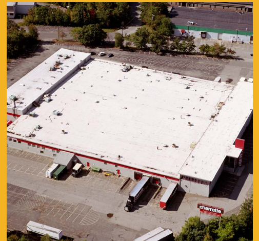
A Sarnafil membrane installed on the Charrette building in Woburn, MA, in 1975, is still performing today.
