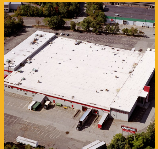
A Sarnafil membrane installed on the Charette building in Woburn, MA, in 1975.
