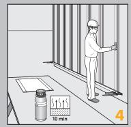
Activate the bond faces with Sika® Aktivator-205. Use a clean, lint-free paper towel and wipe in one direction only (dirty cloths must be replaced).
