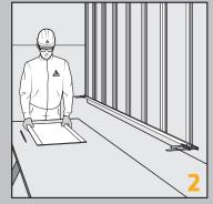
The surface to be bonded must be clean, dry and free from dirt. Abrading with an abrasive pad (80 grit) on the panel and the substructure when recommended for the specific system.
