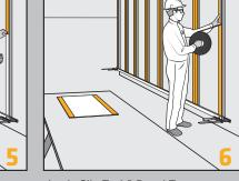
Apply SikaTack® Panel Tape over the whole length of the vertical sections and parallel to the edges.
