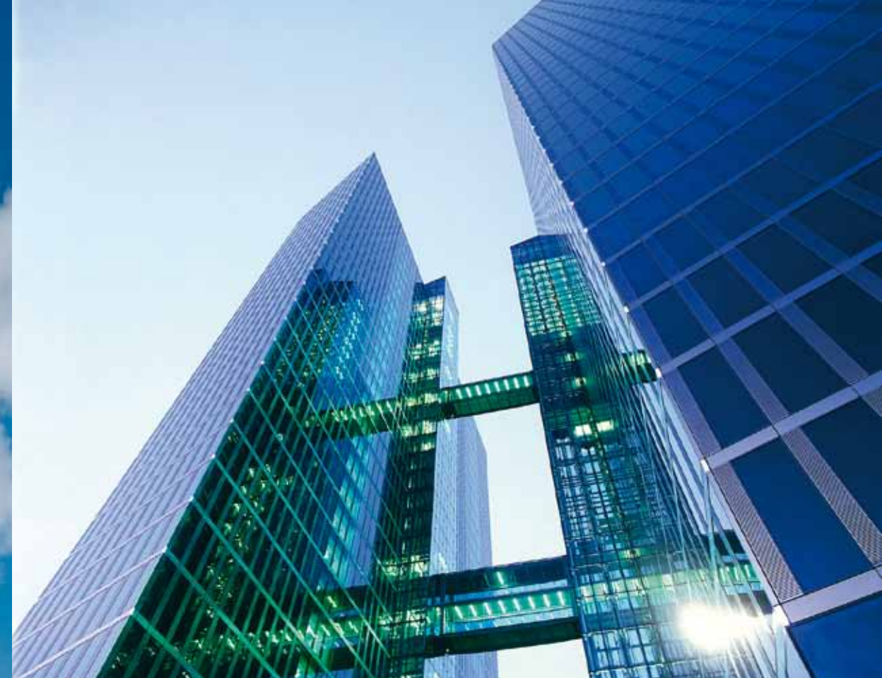
Highlight Towers, Munich, Germany
