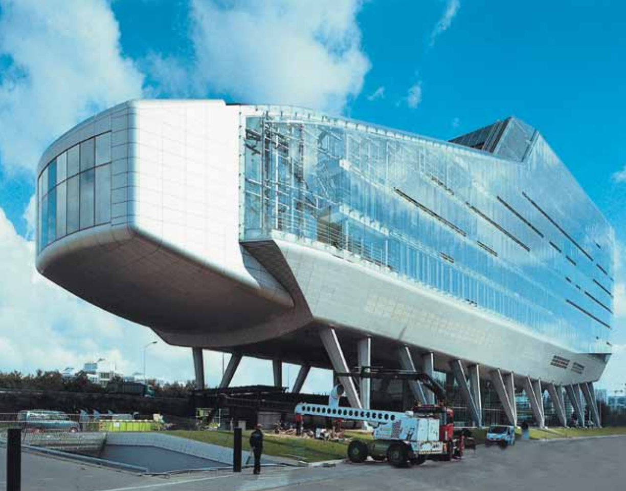
ING Group Headquarters, Amsterdam, Netherlands
