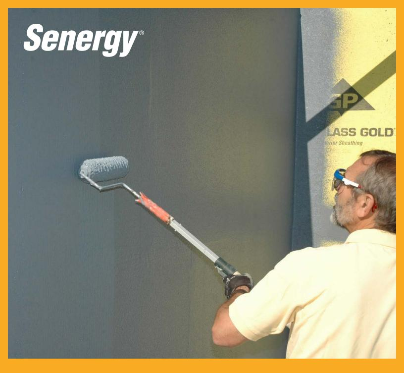
Framed Construction Incorporating Fluid-Applied Senergy Air/Water-Resistive Barriers
