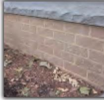
**Description:** 2 1/4" x 7 3/4" bricks with 1/2" mortar joints arranged in running bond pattern.
