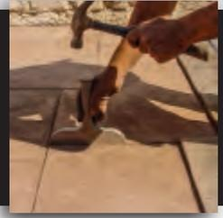
Our tampers, hand chisels and touch-up wheels are a must on every stamping job. The hand chisels and touch-up wheels are used to finish g out lines in difficult eas or on the edges where the stamping mats cannot reach.
