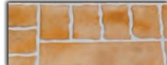
**Description:** Irregular stones varying from 4" x 8" to 5" x 8". Mortar joints from 1/2" to 1". Arranged in single file for borders.
