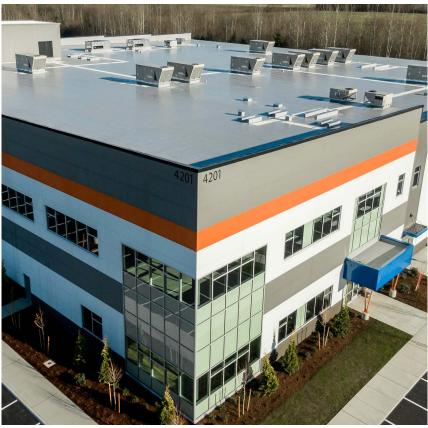
OneDek by All Weather Insulated Panels is a high-performing alternative to traditional multi-layer low slope roof systems. Replacing steel deck and multiple layers of ISO board insulation, a OneDek system requires fewer components and less steps to install, saving construction time, and labor, while providing exceptional energy efficiency for your roof system. An industry exclusive 20-year, full "System Warranty" is provided by Sika Sarnafil.
