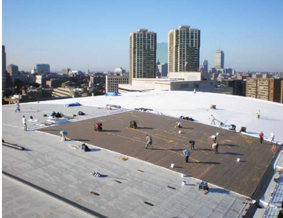
“I love RhinoBond’s speed and ease of installation,” Klein stated. “As soon as you roll out the membrane you can start doing seams right away, which makes the roof watertight much sooner. Our 20-person crew was installing 15,000 to 25,000 square feet of roof a day, which is ten to 15 percent faster than with a mechanically attached system. I try to get most jobs switched to a RhinoBond system.”
