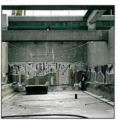
walls, floors, and deck walkways. Petrographic analysis revealed that the deterioration of the concrete was due mainly to corrosion of the rebar which had been accelerated by the lack of sufficient concrete cover.
