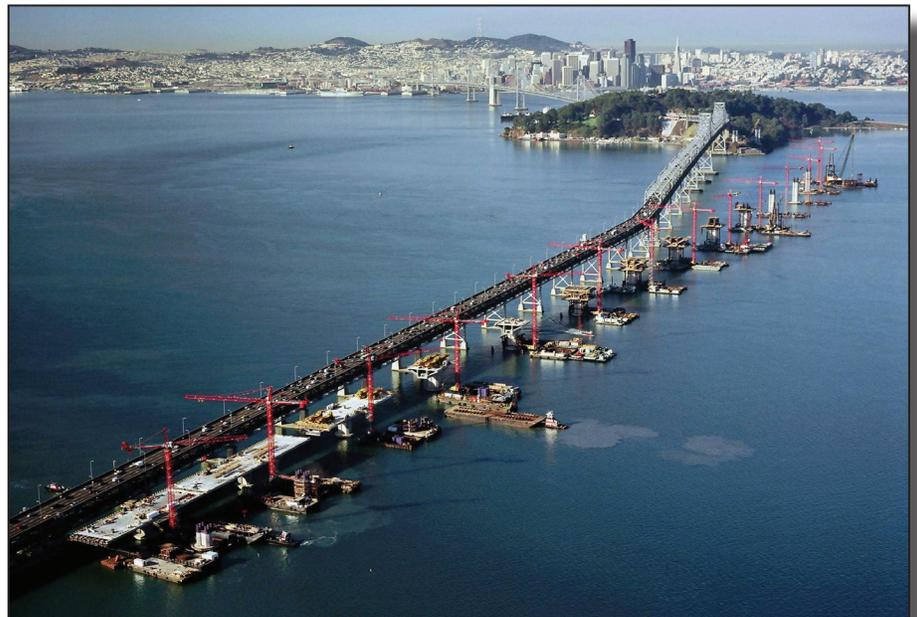
Caltrans' study concluded the western portion connecting San Francisco and Yerba Buena Island could be retrofitted to withstand a major earthquake. They also determined it would be far more cost effective and safer to build a new eastern span rather than retrofit it. The new structure would be designed to meet current seismic codes as well as other codes pertaining to roadway shoulders, lane widths, stopping sight distances and other factors to substantially improve public safety.
