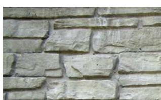
Please note that the #328, #439, #440, #454, #460 (see note #2 below for special instructions), and #477 patterns have special features that result in a finished concrete wall that looks as though it was built using individual stones. This gives the end product a more natural looking appearance. With this in mind, the above patterns do require some special care and attention when being installed in comparison to other plastic formliner patterns that are offered.
