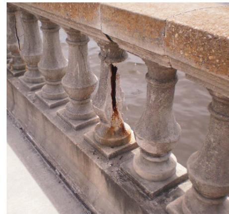
*Damaged baluster revealing reinforced steel.*
