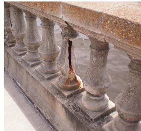
*Damaged baluster revealing reinforced steel.*
