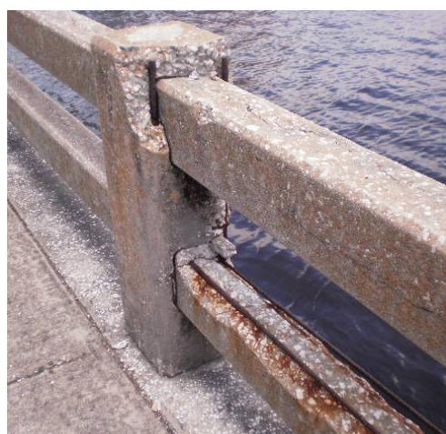
*Damage to a post and rail section.*
