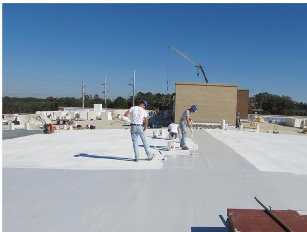
**Sika® Reemat** - a glass fiber matt embedded into Sikalastic® roof coatings for enhanced multi-directional tensile strength. Great for complex details, joints, corners, and protrusions.
