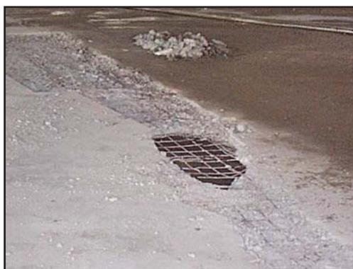
Constructed in the late 60's, this 56,000 square foot Parking Garage consists of conventional cast in place slab and beam construction. Low Concrete cover over the reinforcing steel and exposure to deicing salts had caused corrosion, resulting in extensive cracking and spalling of the concrete. The owner and specifier wanted a long-term repair and protection solution to prevent further deterioration of the concrete in this structure extending the service life of the garage.
