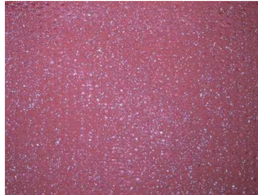
Insufficient broadcast of sand
