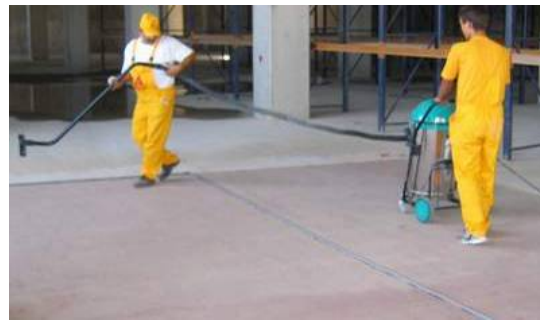
Bare spots as can be seen above, can cause lack of bonding of the screed, and possibly the formation of cracks as a consequence.
