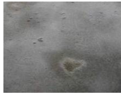
Bare spots as can be seen above, can cause lack of bonding of the screed, and possibly the formation of cracks as a consequence.
