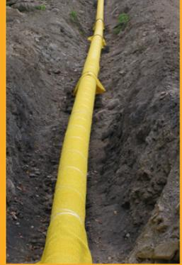
**ROLLS:** Sized to match any pipeline diameter up to 22".
