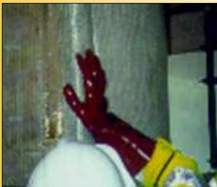
**3** Wet fabric is laid-up onto primed concrete surface
