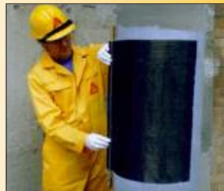
**2** Dry fabric is laid-up directly onto the saturated concrete surface
