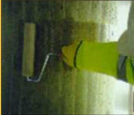
**1** Priming the concrete with Sikadur epoxy resin
