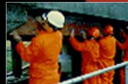
Shear strengthening of concrete bridge beam with steel plates and special Sikadur epoxy.
