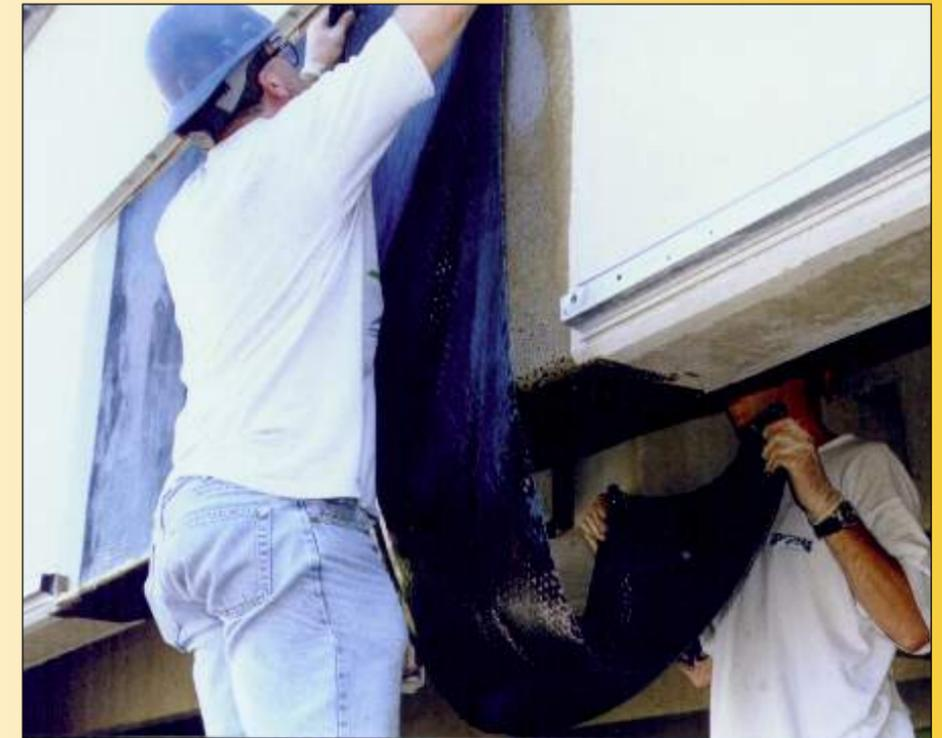
*Shear strengthening of spandrel beam with CFRP fabric.*
