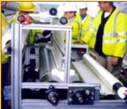
**2** Impregnation of fabric using saturator machine
