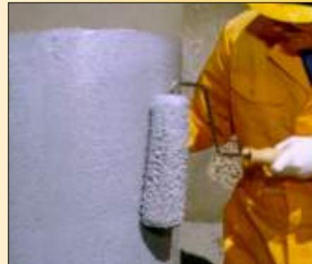
**1** Priming and saturating the concrete with Sikadur epoxy resin
