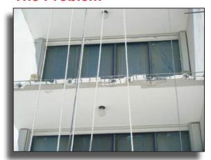
The Waterside Tower Condominium is a 10 story building located in the coastal area of Miami, Florida. The 118 unit high-rise building was constructed in 1972 with post-tensioned concrete. After 30 years of the highly corrosive environment of South Florida the building started to show signs of deterioration. The most evident sign of failure was at the balcony slab edge.
