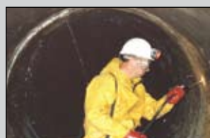
Chemical Grouts Expanding, polyethylene chemical grout used to stop leaks
