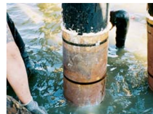
Repaired Pile with Epoxy Mortar
