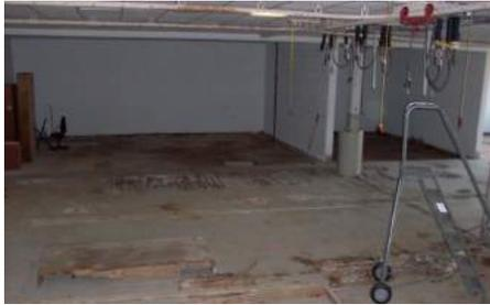
Top side spalling and steel corrosion.
