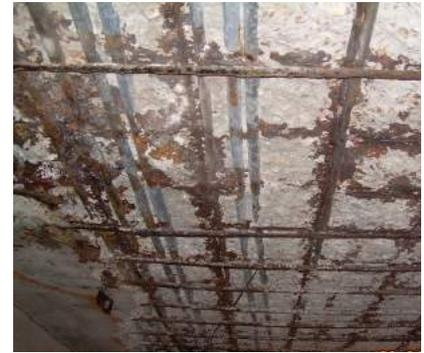
Underside spalling and steel corrosion.
