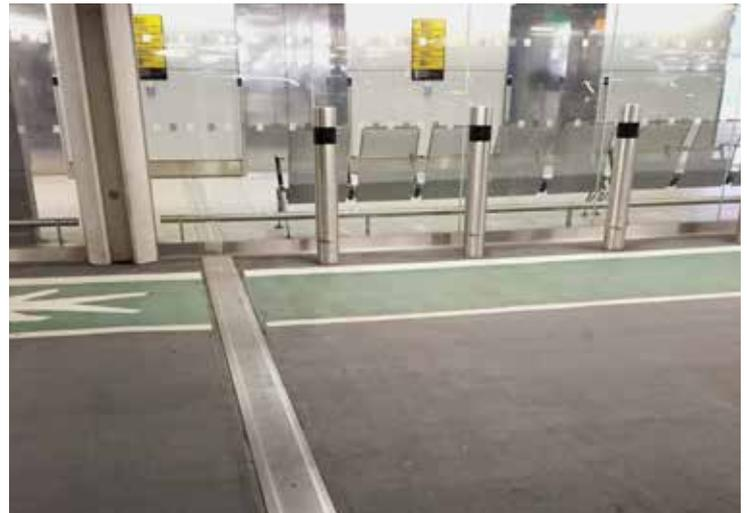
Sikafloor® and Sika® Emseal movement joints working together as a complete system.
