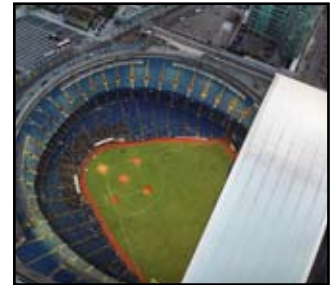
Canada's Skydome roof system was installed in 1989 and is still in service.
