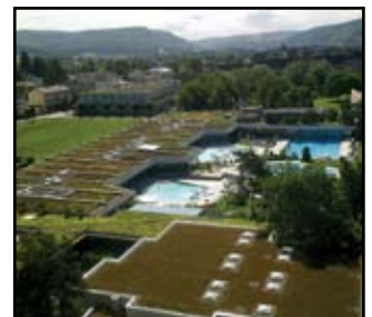
The first Sarnafil green roof was installed in 1969 and is still in place.
