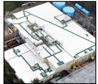
The EnergySmart Roof has a history of high performance and longevity.
