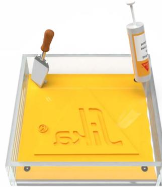
**2** Seal all formliner joints, tie holes, and penetrations created by mechanical fasteners using neutral cure silicone sealant.
