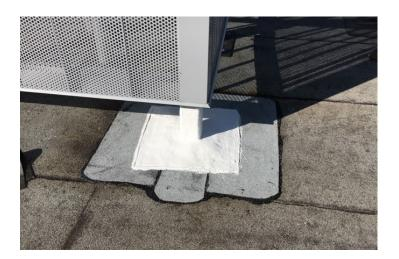
In addition to the work on the parapets the Sikalastic® RoofPro system was ideallly suited for reworking some of the flashings penetrating the area of existing BUR roof that was not replaced. Stone roofing having worked with both PMMA resins and Sikalastic®-641 Lo VOC chose to use Sikalastic®-641 Lo VOC for this application due to its very user friendly characteristics.
