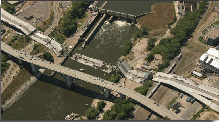
deck truss construction while all but two of the eleven approach spans were steel multi-girder construction, the two exceptions being concrete slab construction. The bridge ranked as Minnesota’s fifth busiest and carried more than 140,000 vehicles a day. It was estimated that the loss of the bridge resulted in \$400,000 per day in lost revenue, increased commuter expenses and stress on surrounding roads.
